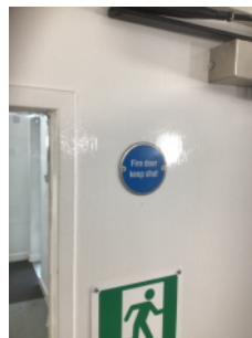
“Fire Door Keep Shut” signage on staircase doors
