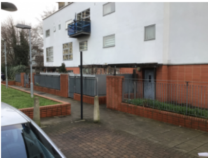
57-63 De Beauvoir Crescent, direct external access, ground floor, side
