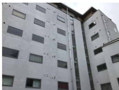
External walls - rear elevation
