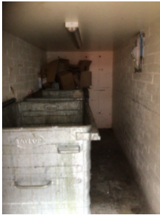
Externally accessed bin store
