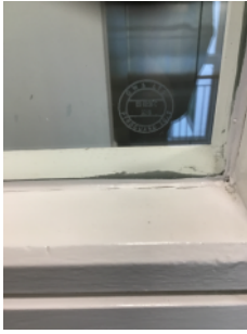
Acid etching on “Pyroguard” FR Glazed lobbies.
