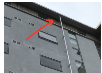
Timber cladding on the sixth floor.
