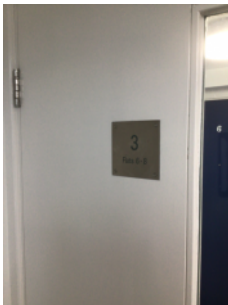
Floor numbers are clearly identified
