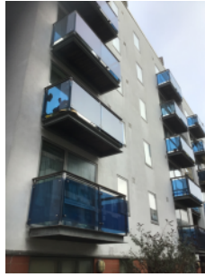
Configuration and construction of private balconies
