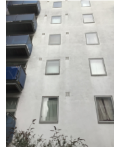
External walls-front elevation
