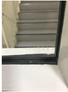
Acid etching on glazing.
