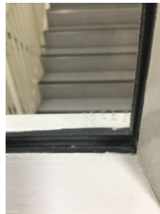
Acid etching on glazing.
