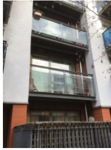
Timber cladding within inset (Juliet) balconies
