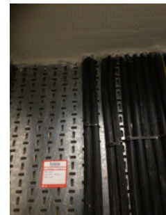
Fire stopping in risers
