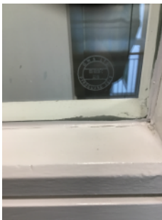
Acid etching on “Pyroguard” FR Glazed lobbies.
