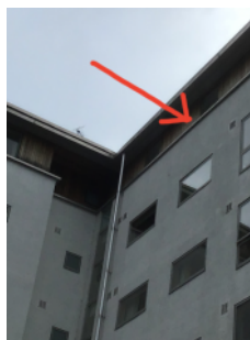
Timber cladding on sixth floor
