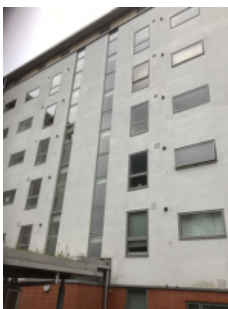
External walls end rear elevation
