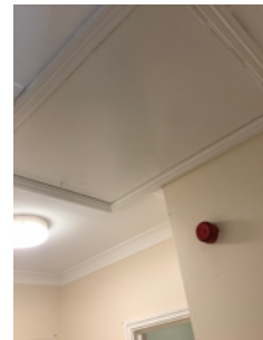
It was not possible to access loft hatches and roof spaces
