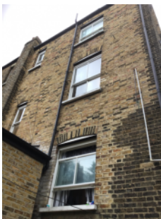
External walls, rear of building
