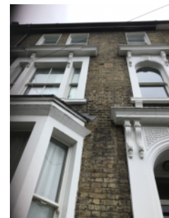
External Walls, front of building
