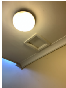
It was not possible to access loft hatches and roof spaces
