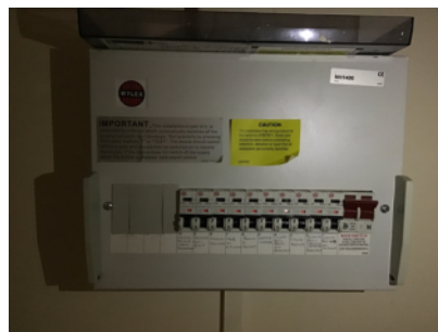
Consumer unit in No.20A, no test label
