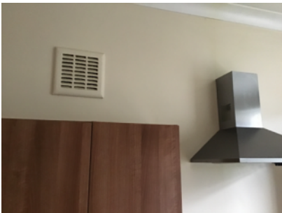
Wall vent in kitchen, to open air
