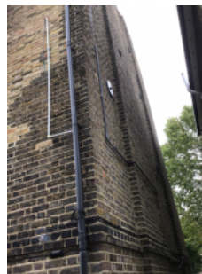
External walls, side of building
