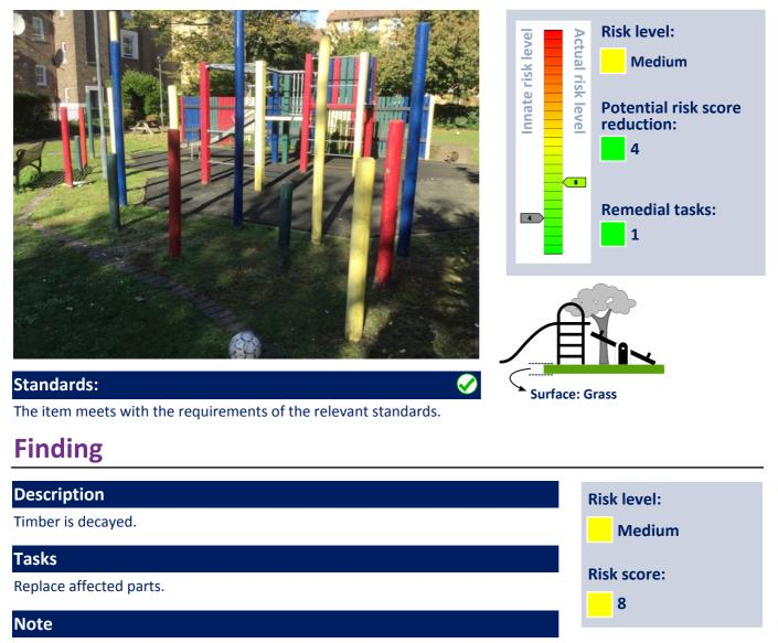
Posts decayed at ground level one post snapped off at ground level - replace.
