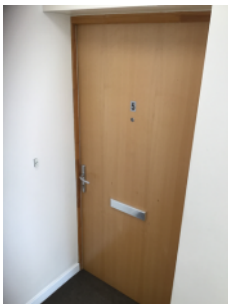
Example of typical flat entrance door in the building
