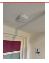
**ISSUE 4 SMOKE DETECTOR.** First floor detector tested sounded.
