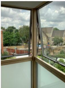
Openable windows in the staircase
