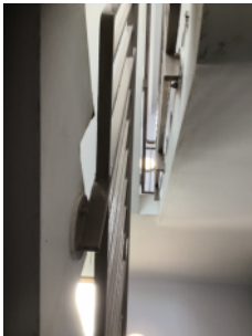
Photo showing concrete floors and stairs
