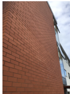
External walls, part brick, part rendered.
