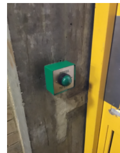
Exit device provided on main entrance door.
