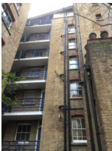
Brick/mortar external walls - rear elevation
