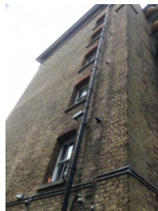
External walls – side elevation.
