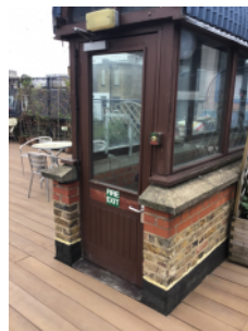
Alternative exit route on roof, through to neighbouring Thurston building.
