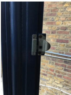
Window fastenings - not standard sized key
