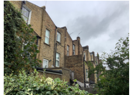
Brick/mortar external walls at rear of the terrace
