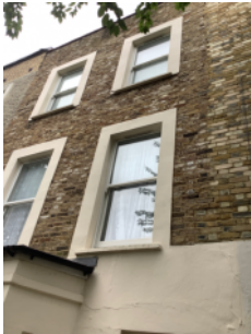
Brick/mortar external walls
