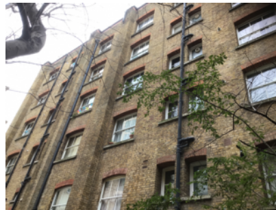
External walls-rear elevation.
