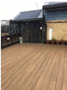
Alternative exit route through to neighbouring Holland building.
