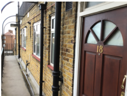
Fanlights and window glazing located above 1.1m
