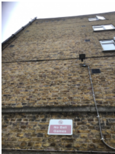
Original brick/mortar external walls
