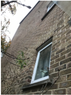
External walls of brick/mortar construction.
