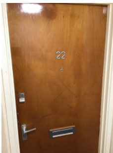
Original flat entrance door.
