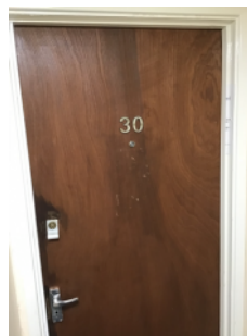
Replacement timber flat entrance door
