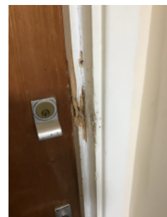
Damaged doorframe
