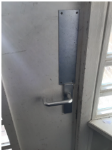
Final exit door from staircase
