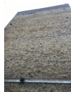
Original brick/mortar wall construction
