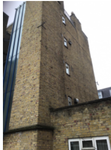
Original brick/mortar walls
