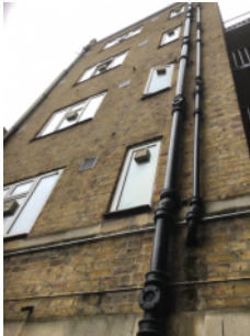
Original brick/mortar walls.
