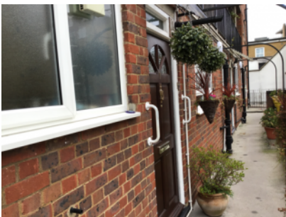
Windows, fanlights and vision panels above 1.1m
