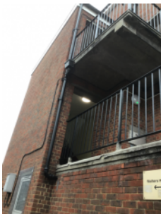
Brick/mortar external walls
