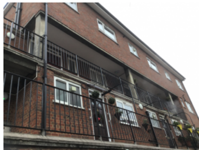
Brick/mortar external walls
