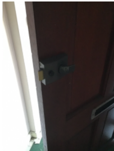
The main entrance door has a lever operated lock.
