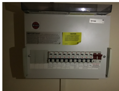
Consumer unit in No.20A, no test label
