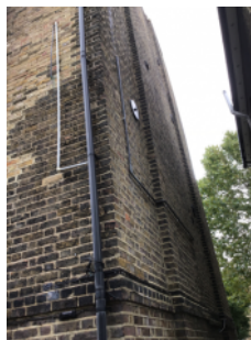
External walls, side of building
