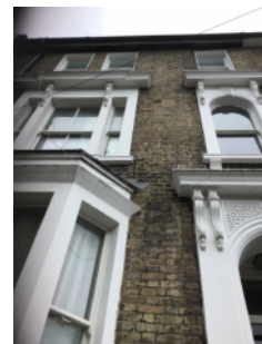
External Walls, front of building
