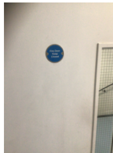
“Fire door keep closed” signage on staircase doors
