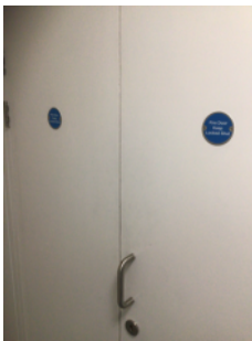
“Fire door keep locked shut” signage on riser cupboard doors
