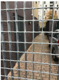
Main gas meter store
