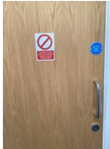
Riser cupboard door signage
