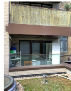
Combustibles on private balconies
