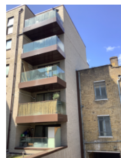
External walls with private balconies - rear of building
