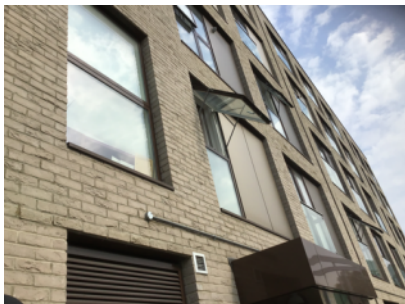
FRONT OF BUILDING : Visual inspection only - Brick external wall system
