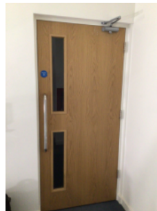
Staircase lobby door
