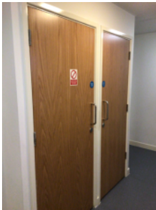
Riser cupboard doors
