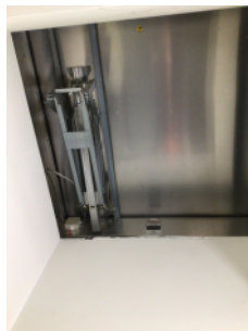
Head of staircase AOV
