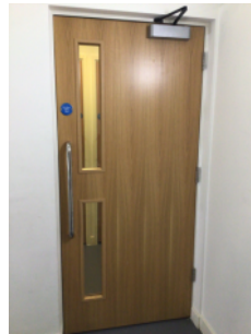
Staircase lobby door
