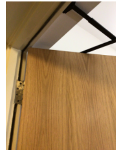
Self closer with intumescent strips and seals
