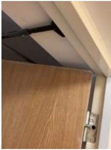
Example of flat entrance door
