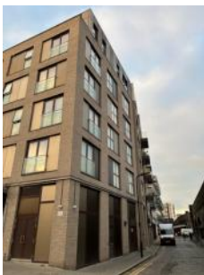
Side aspect of building
