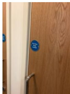
Riser cupboard door signage
