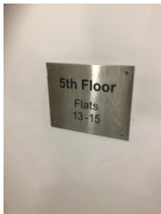
The building floor numbers are clearly identified on each floor landing
