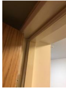
Example of believed surface mounted smoke seal (photo from 1 Dunston Rd)
