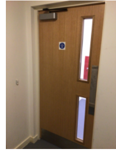
Staircase lobby door
