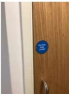
Riser cupboard door signage
