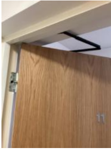
Typical flat entry door
