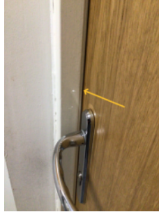
Possible surface mounted smoke seal
