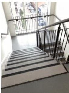
Clear escape route with contrasting stair nosings.
