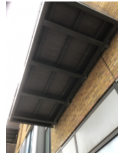
Underside of private balconies
