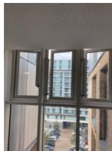
Lift lobby AOV
