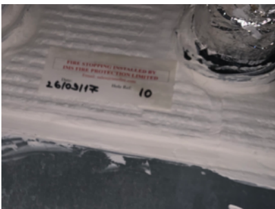
Example of fire stopping certification label - IMS Fire Protection Ltd 2017
