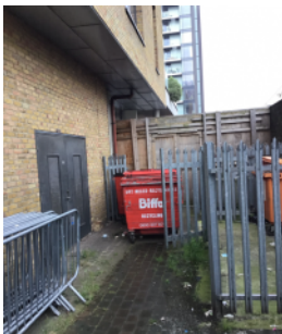
Wheelie bins under overhang.
