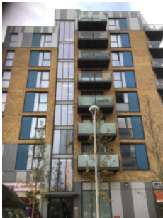
Front elevation - showing private balconies and cladded EWS to 7th floor
