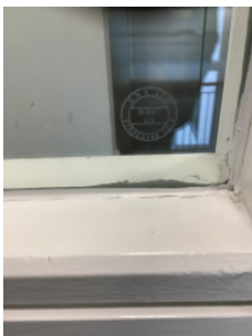
Acid etching on “Pyroguard” FR Glazed lobbies.
