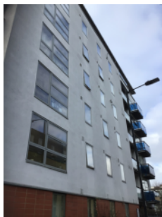
External walls-end elevation, also showing private balconies on this elevation.
