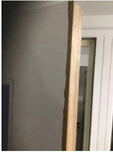
Hardwood door lipping fitted to staircase doors.
