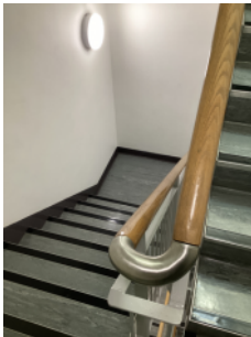
Escape route with contrasting stair nosings
