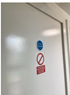
Riser cupboard door signage
