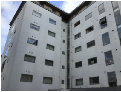
External walls - rear elevation
