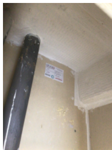
Fire stopping within riser cupboards
