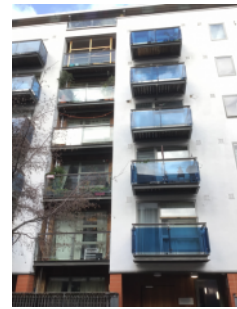
External walls – front elevation
