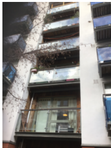
Timber cladding on the inside of (Juliet) private balcony
