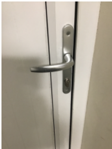
Door furniture on main entrance door and rear door.
