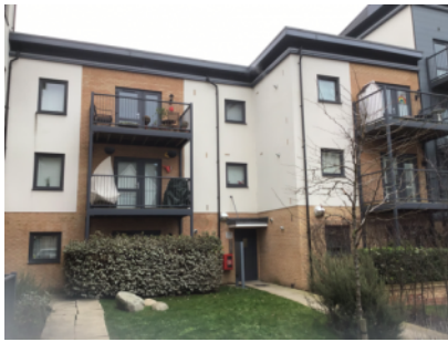
Front elevation- brick/mortar construction with rendered section
