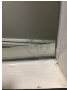
Acid Etching on FR Glazing in staircase doors - Pyrocet XP - BS476, EN12150
