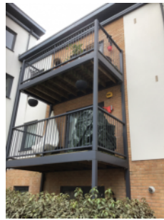
Private balconies located on the front elevation
