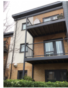
Private balconies located on the front elevation
