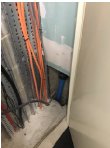
Access cut into lining of cupboard on 1st floor.
