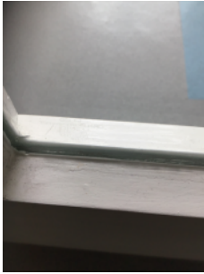
Acid etching (pyrogard) on glazing installed in lobby doors.
