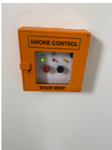
Manual smoke control devices
