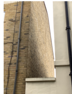
Brick/mortar external walls- end elevation
