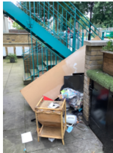
Unsecured Combustible items within the curtilage of the building
