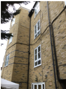
REAR ELEVATION: Brick external walls.
