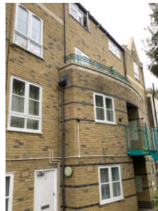
FRONT ELEVATION: brick external walls
