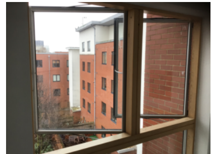
Window AOVs in corridors (3rd floor)
