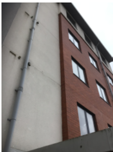
External walls – rear elevation
