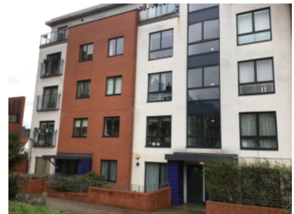
External walls - front elevation
