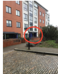
Proximity of main entrance door from closest point of fire appliance access
