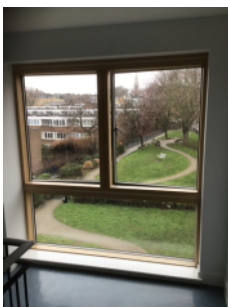
Openable windows in the staircase - first second and third floors
