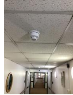
BS5839-1 detector and sounder in corridor
