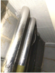
Fire stopping within riser cupboards
