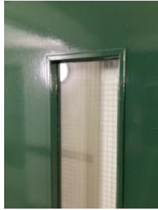
Georgian wired glazing in cross corridor door
