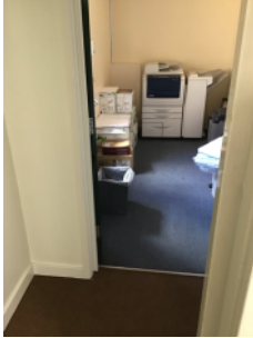
Obstructed fire door
