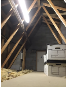
Compartmentation in roof space
