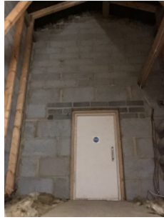
Compartmentation in roof space
