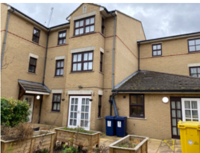
Rear elevation of the building.
