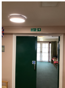
Escape route signage
