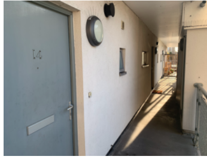
Showing window glazing to flats - above 1.1m
