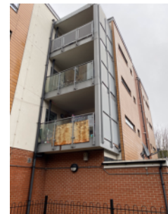
Private balconies on rear elevation.
