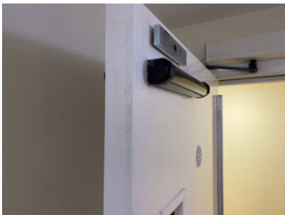
FD60S SC Doors installed in the staircase.
