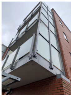
Photograph showing construction of private balconies.
