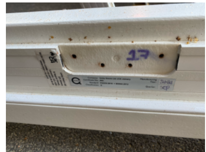
BMTrada QMARK certification label on NEW door frames being installed
