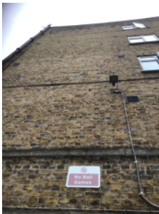
Original brick/mortar external walls
