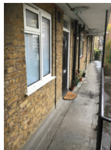
All glazing on common balconies above 1.1m
