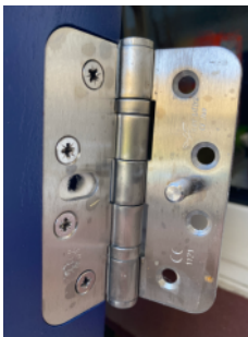
Fire rated hinges on the new door sets being installed
