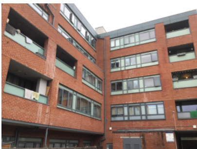
Brick/ mortar external walls with glazed panels
