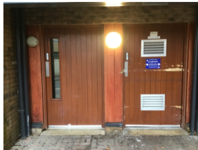
Access to basement carpark (left), and refuse store (right)
