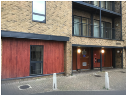
Ground floor partially timber clad
