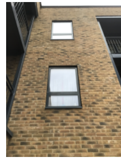
Brick/mortar external walls to ground, 1st , 2nd and 3rd floors
