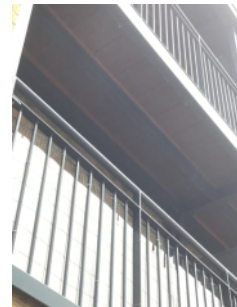
Private balconies-steel framed with timber deck
