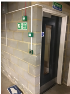
Exit from basement carpark
