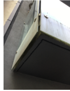
Common balconies- Concrete base with glazed up-stands
