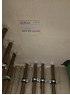
Example of installed fire stopping in riser cupboards.
