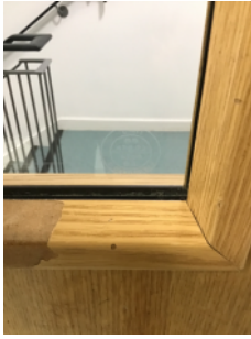
Acid etching on staircase door glazing
