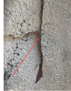
Showing insulated material beneath rendered surface.
