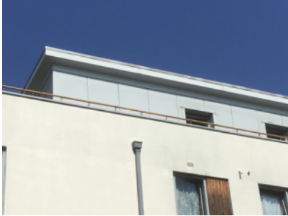
Cladded external wall system installed on fourth floor.
