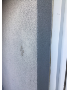
Rendered external wall surface
