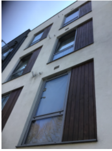
Timber rain screens around windows.
