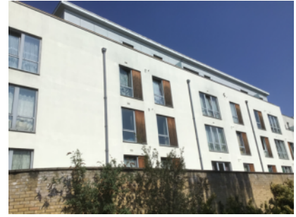
External walls – rear elevation
