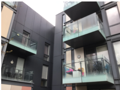
External walls with balconies rear elevation
