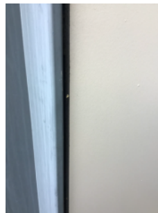
Cladding to building exterior which is a composite boarding - not ACM
