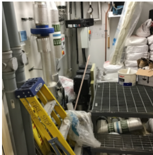
Ground floor plant room being used as a store
