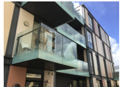
External walls - front elevation
