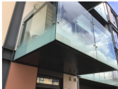
Construction of private balconies
