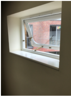
Openable windows in staircase
