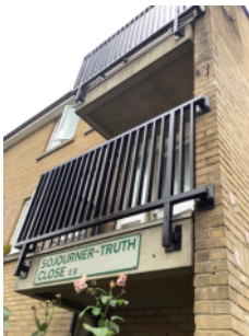
Construction of private balconies
