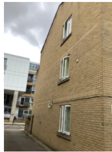
Brick/mortar external walls, - end elevation
