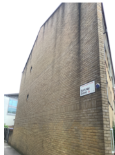
Brick/mortar external walls - end elevation
