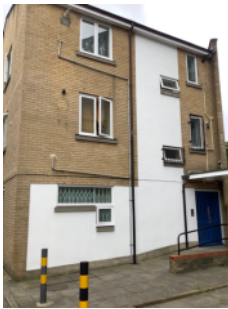
Brick/mortar external walls, with rendered section - front elevation
