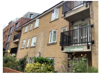
Brick/mortar external walls, with rendered section - rear elevation
