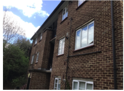
Brick/Mortar External walls - rear elevation
