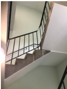
Concrete walls, stairs and floors in the building.
