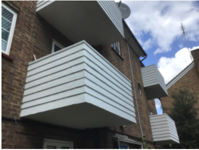
Concrete balcony decks with concrete up stands
