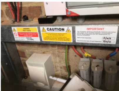
Evidence of testing of fixed electrical installations
