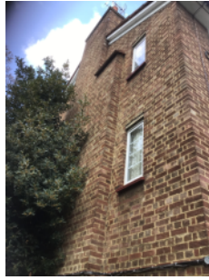
Brick/Mortar External walls - end elevation
