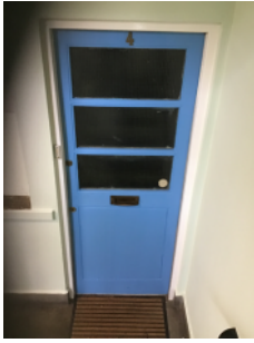
Example of flat entrance doors provided in the building.
