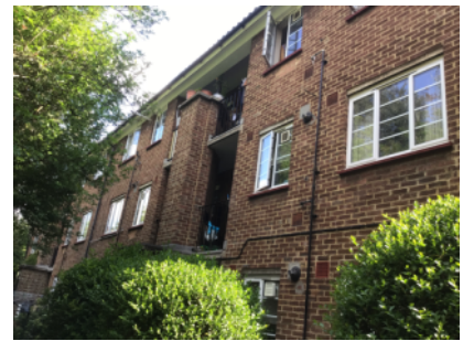
Brick/mortar construction, external walls, rear elevation
