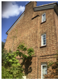
Brick/mortar construction, external walls, end elevation
