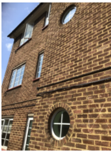
Brick/mortar construction, external walls, front elevation
