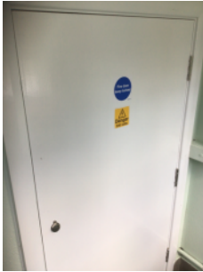
Fire door keep locked signage on electrical cupboard door.
