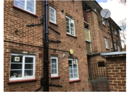
Brick/mortar external walls – rear elevation
