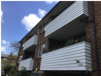
Private balconies on the front elevation of the building.
