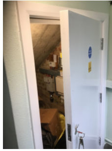
New FD30S door fitted to the electrical cupboard.
