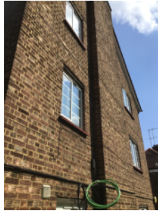
Brick/mortar external walls – end elevation
