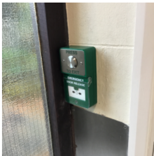
Exit release mechanism
