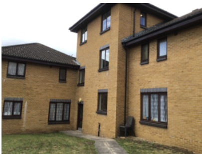
Brick external walls to the rear of the building
