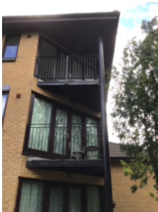
Steel balconies with steel decks
