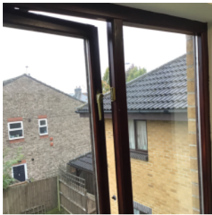
Openable windows in staircase
