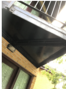
Steel deck of balconies
