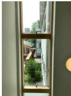
Openable windows in the staircase.
