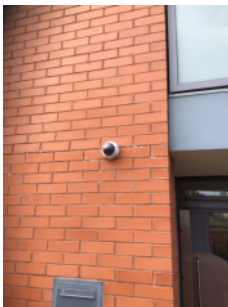
External CCTV Camera
