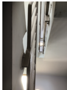
Photo showing concrete floors and stairs
