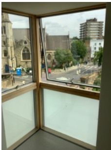
Openable windows in the staircase.
