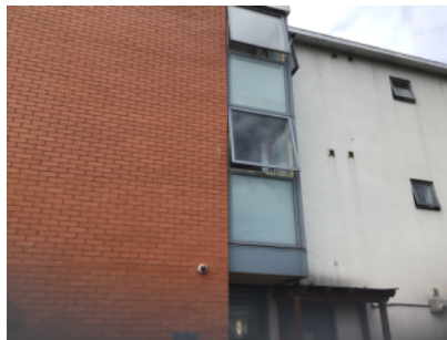
External walls, part brick, part rendered.
