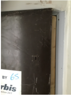
Security door fitted to entrance of Void flat (6).
