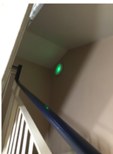
Maintained emergency lighting is provided
