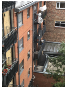
External walls, rear of building.
