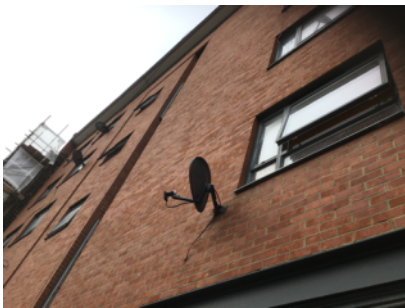
Brick walls to front face of building
