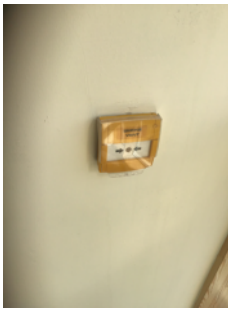
Smoke vent manual actuation
