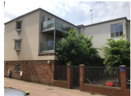
External walls, rear elevation
