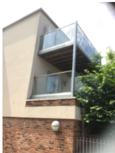
Only two private balconies are provided at rear of building
