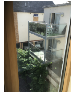
Balconies generally clear of combustibles
