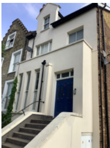
External walls, front elevation
