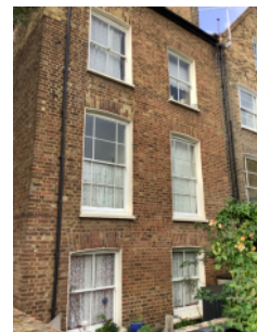
External walls, rear elevation
