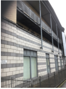
External walls-front elevation
