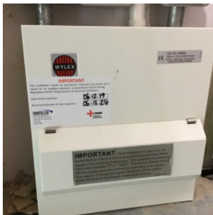
Evidence of EIC inspection in date
