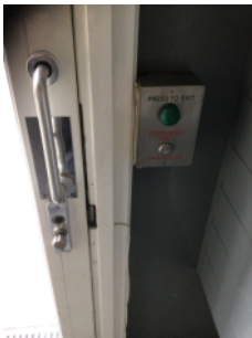
Electromagnetic door release mechanism with emergency override.
