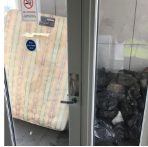
Combustibles in escape route
