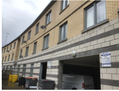
External walls – rear elevation
