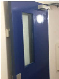
Georgian wired glazing installed in corridor doors.
