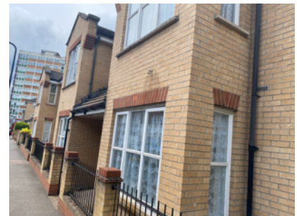
External walls - front elevation.
